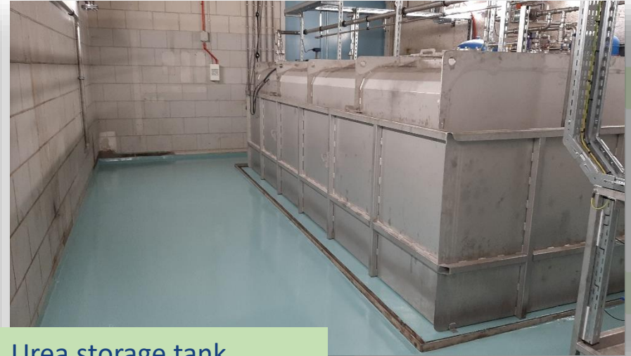
Urea storage tank
