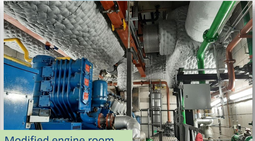
Modified engine room
