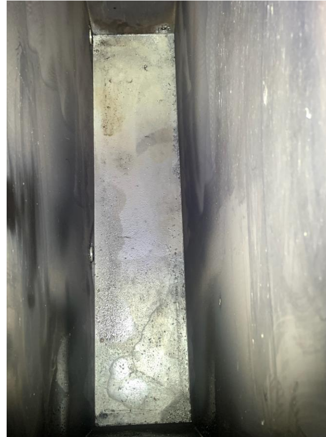
Tank after Power Washing
