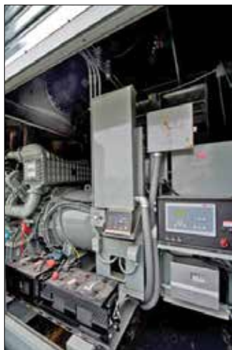
MTU Onsite Energy Series 4000 generator sets are approved for an 85 percent 24-hour average load factor (15 percent above industry standard).
