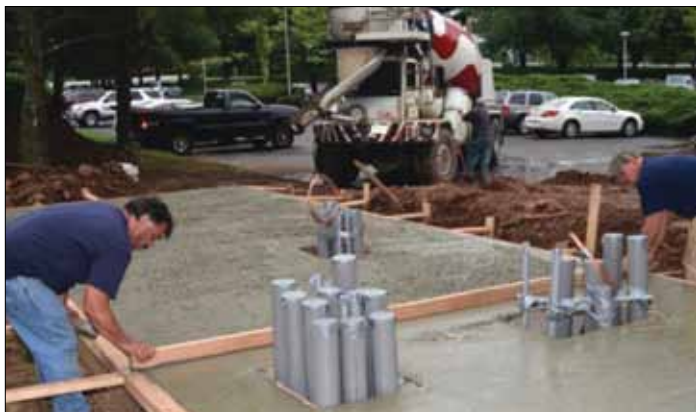
Building the pad.
