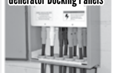
Generator Docking Panels
