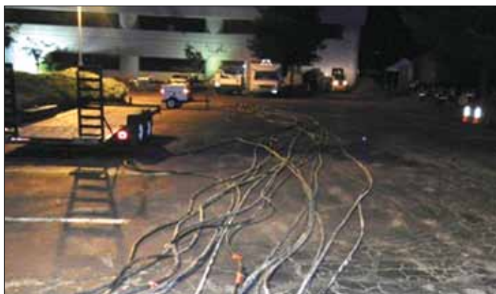
The work does not stop at sundown.
