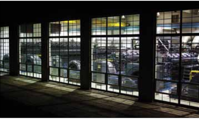
Today, FME continues to bring power to places where it is needed most. Shown here is a photo of an Opposed-Piston and Colt Pielstick power installation located in Goodland, Kansas.
