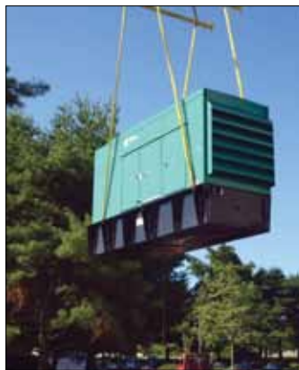
Installing the generator set.
