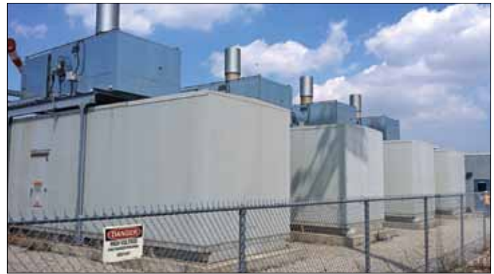
Figure 4: Example of Selective Catalytic Reduction System with Integral Silencing
