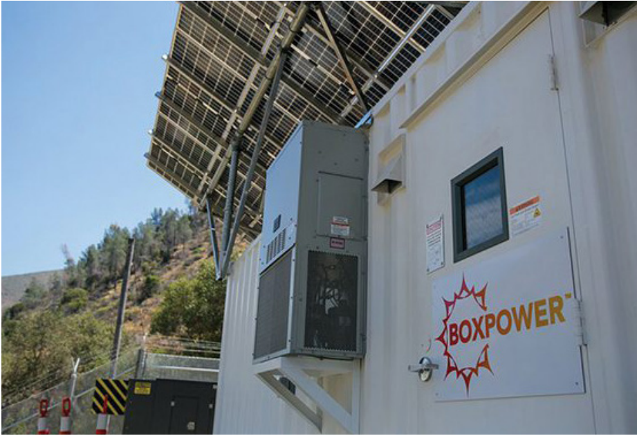
2. BoxPower SolarContainer with container-mounted solar array in Briceburg, California. The SolarContainer also includes a 27.2-kW/68.4-kWh lithium ferro phosphate battery energy storage system. Courtesy: BoxPower
